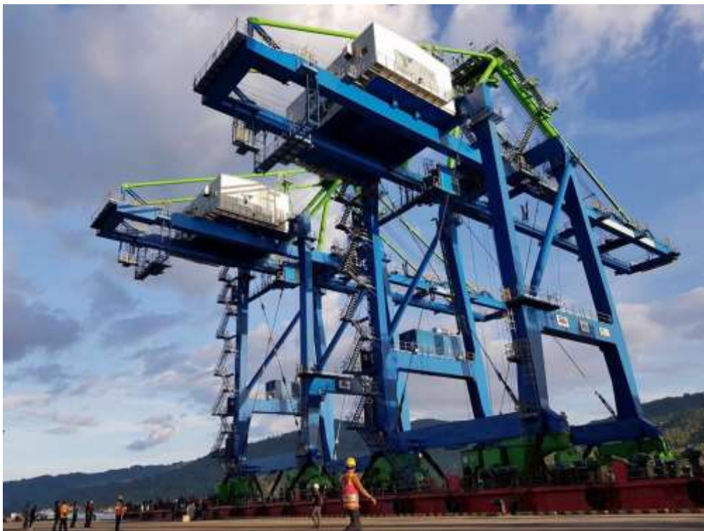
1500kva genset for STS of Pelindo 4
