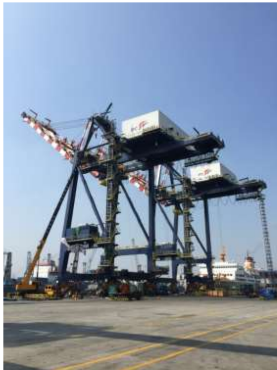
1600kva genset for STS of Pelindo 2
