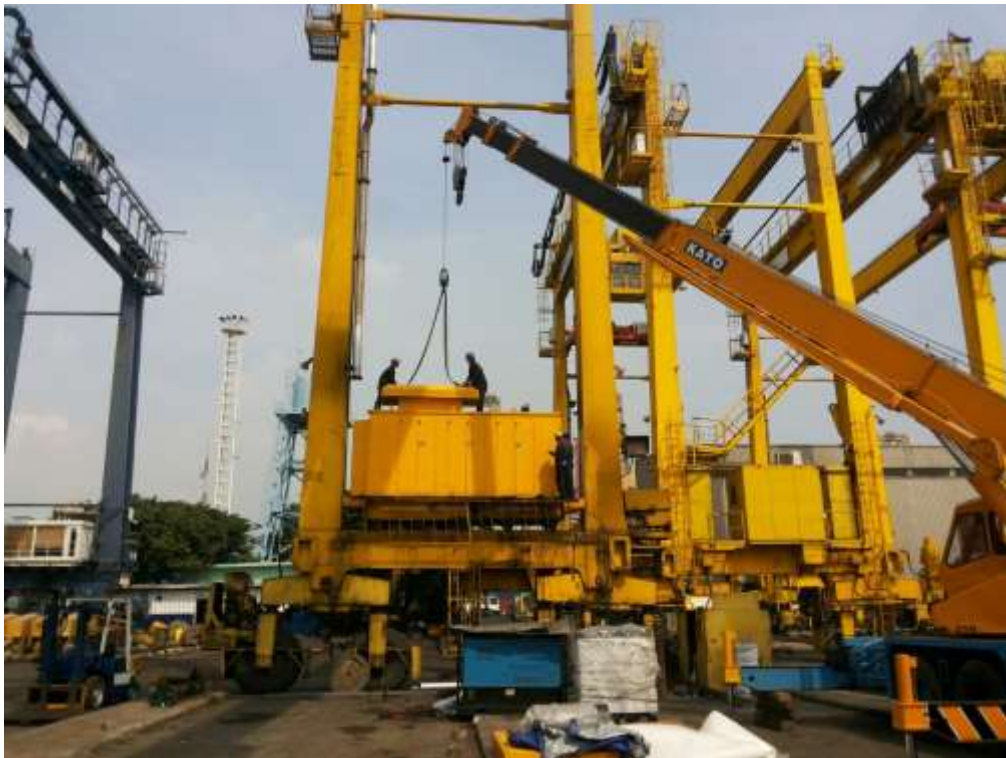
500kva genset replacement for RTG of JICT
